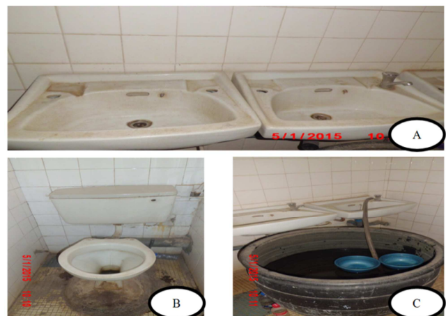
Figure 1. Water supply, sanitary and handwashing facility at Oladele Ajose Building: A-Handwashing facilities; B-Sanitation facility and C-Water supply system.
