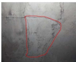
Figure 8. Lining cracks around the hole at arch crown.
