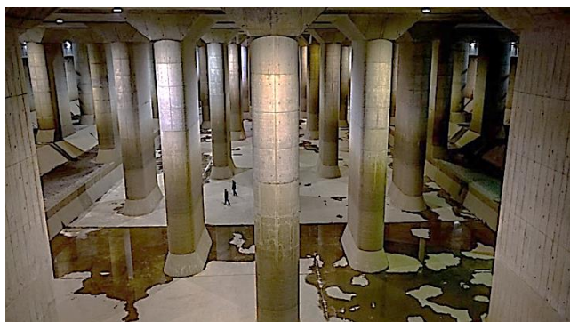
Figure 3. Tokyo underground drainage system - water pressure control bath (size 178x77x18 meters).
