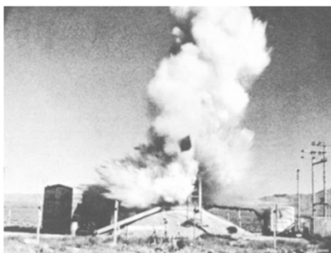
Figure 20. Borax-I criticality and explosion test in 1955 resulted in a much larger explosion than expected due to previously unknown hydrogen explosion effects (McLaughlin, et al. [49]).
