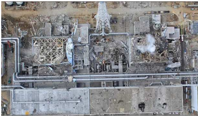
Figure 1. Preventable Fukushima explosions and fire damages following a tsunami, meltdown, and water hammer (NRC.gov).
