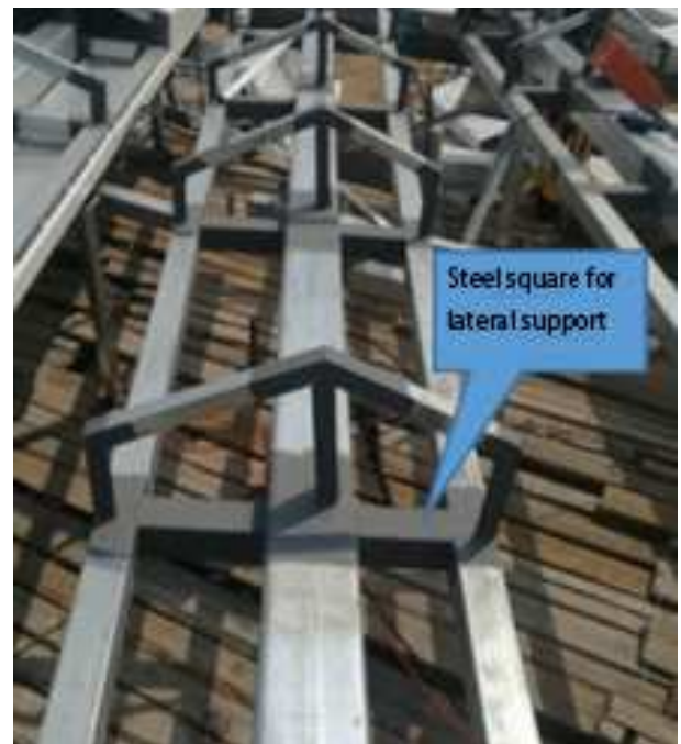
Figure 15. Completion of steel truss.
