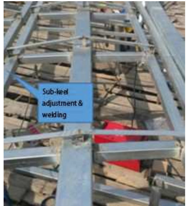
Figure 14. Installation of fixing angle steel of aluminum plate.
