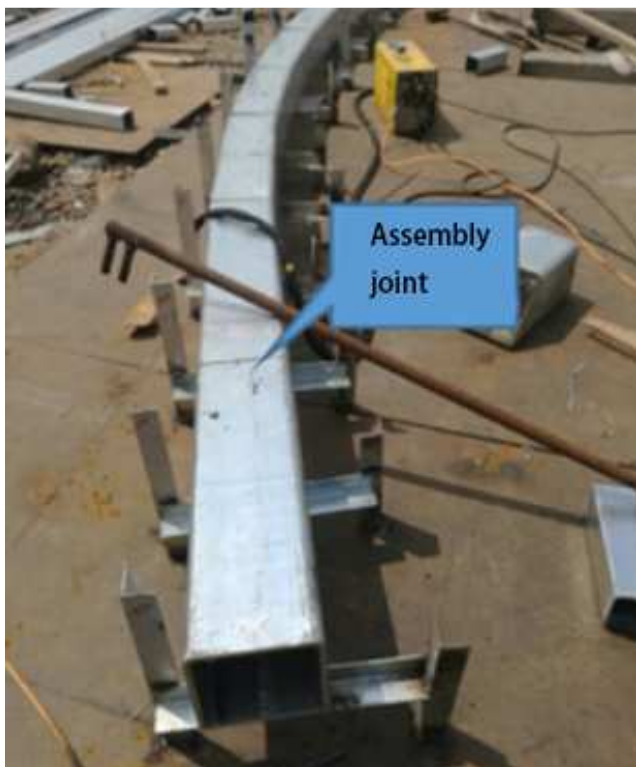
Figure 8. Steel tube assembly.
