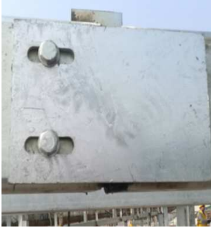
Figure 11. Steel truss square connection.
