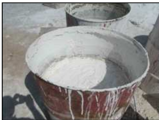
Figure 3. Keeping lime in open environment after slaking.
