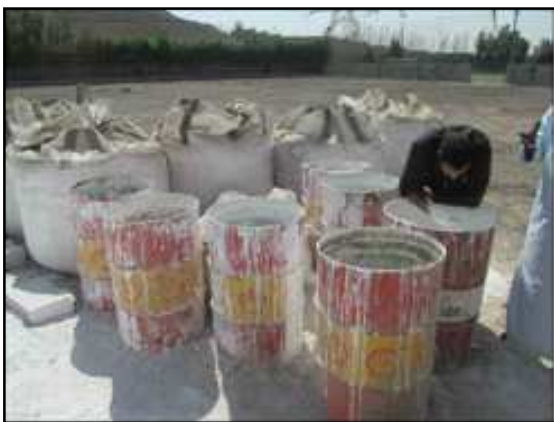
Figure 2. Slaking lime in metal barrels without covering.
