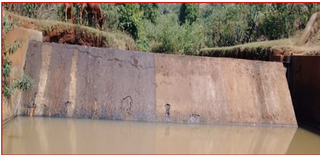
Figure 7. Lack of under sluice gate.
