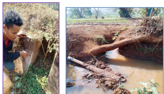
Figure 10. Clogging of turnout structure.
