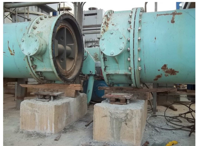
Figure 2. Modification of 3B CW pump discharge piping system.
