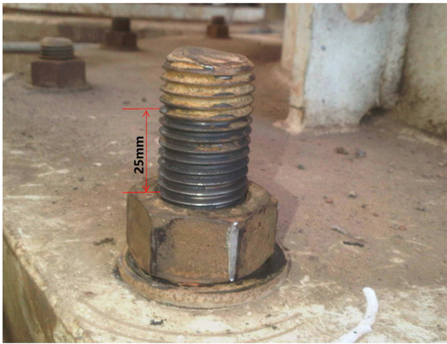
Figure 3. One anchor bolt of 3B drawn out.
