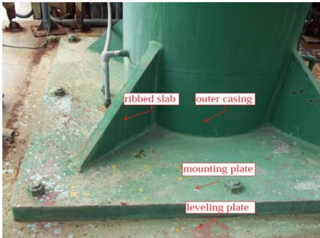
Figure 5. Outer casing and mounting plate of circulating water pump in phase I.
