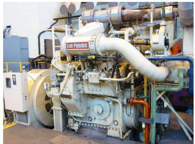
Figure 1. Coal Fueled Diesel Power Plant (6 MW): a - A typical Coal Diesel System with a single 6 MW engine, b - Test Engine Area [8].
