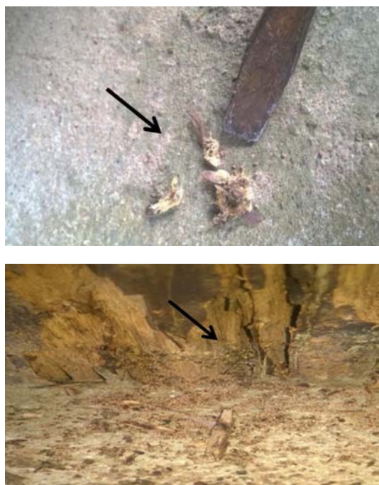
Figure 3. Wing termite and head of worker termite died at position of wooden pillar at house on stilts of Tan Da Resort.
